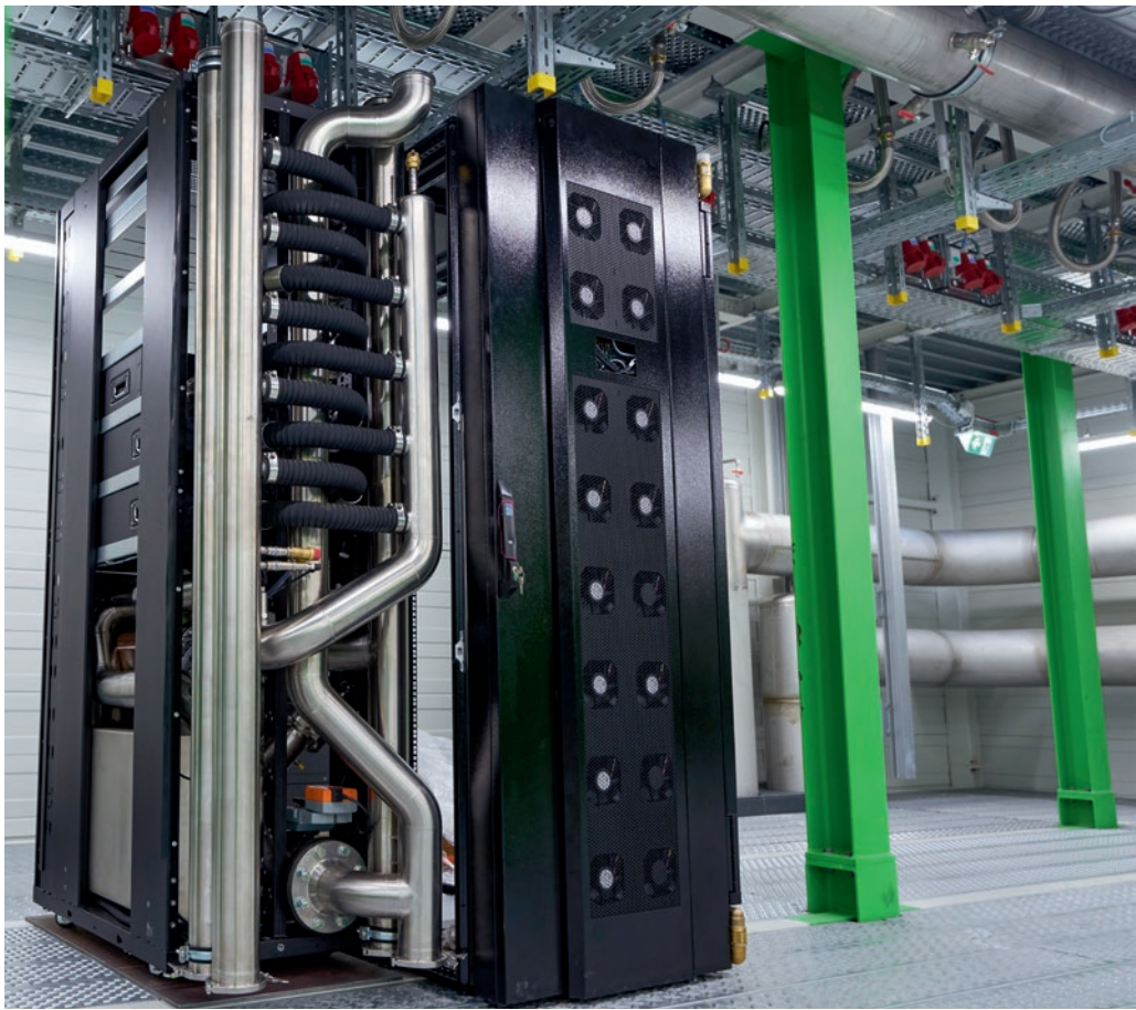
Power in the tightest of spaces – a cooling output of over 1 MW for direct chip cooling with water.
